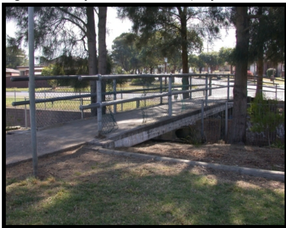
Figure 9- Parry Park, Lakemba (City of Canterbury, 2011)
