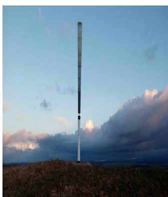
Figure 4. Prototype of Bladeless wind turbines, Spain [9][12]
