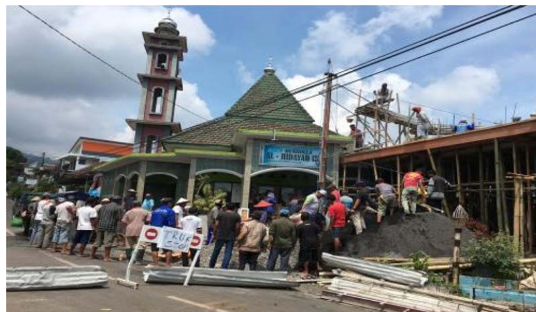
Figure 1. Soyo in building a mosque
