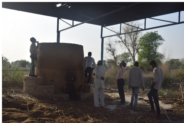
Figure 6. Inspection of newly developed kilns at the installation site
