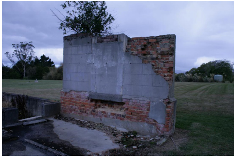
Figure 3 Building remnants at Seacliff Asylum, Truby King Reserve, Otago, New Zealand. Photograph by author, April 2010.
