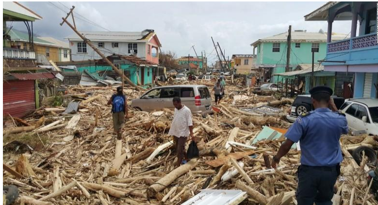
Figure 2: Devastation of Roseau's buildings and infrastructure after Hurricane Maria struck Dominica in 2017
