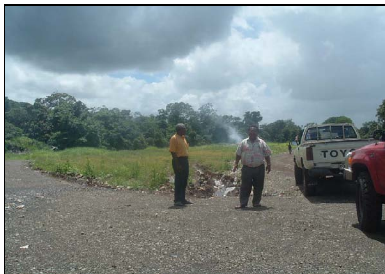
The Mayor and Town Manager inspect the reconstructed road to the dump
