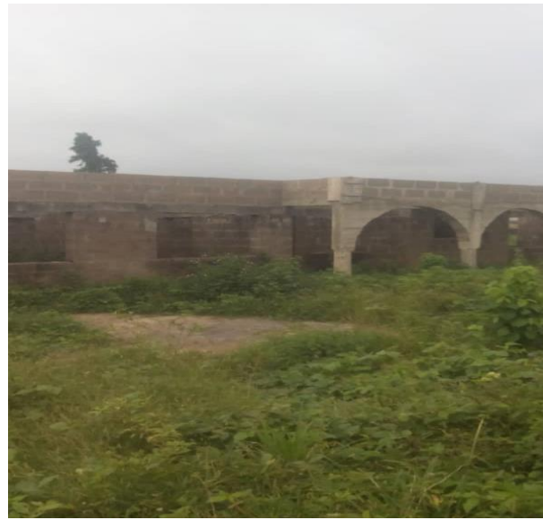
Figure 6: Health facility under construction
