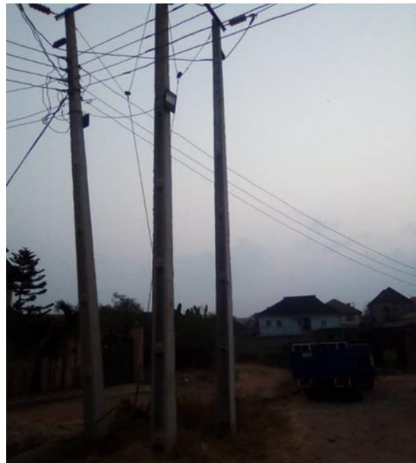
Figure 4: Installed electric poles and cables
