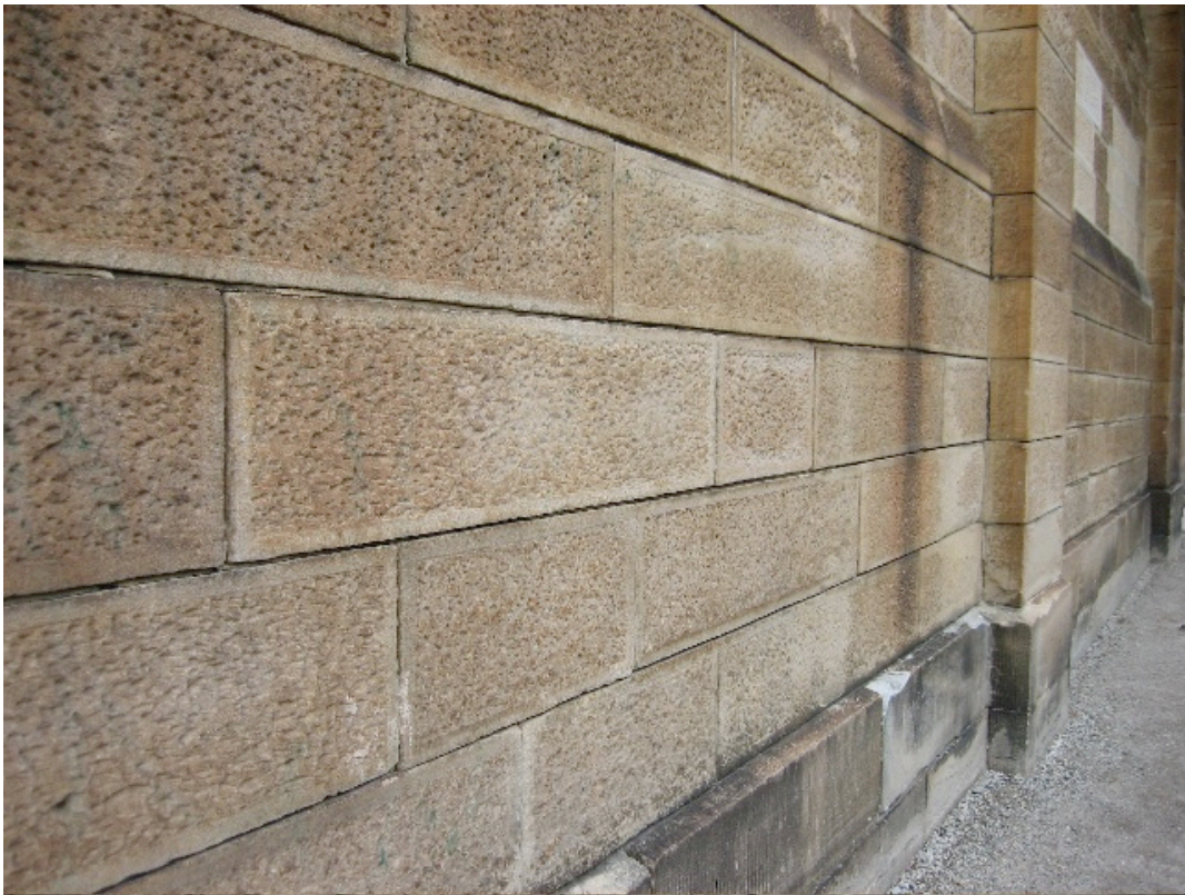
Sandstone wall, National Art School, 2007 (photograph: Jan Idle)
