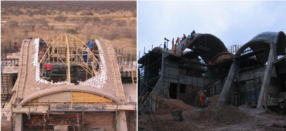
Figure 2 Corrections taken, construction progressed in different sections
