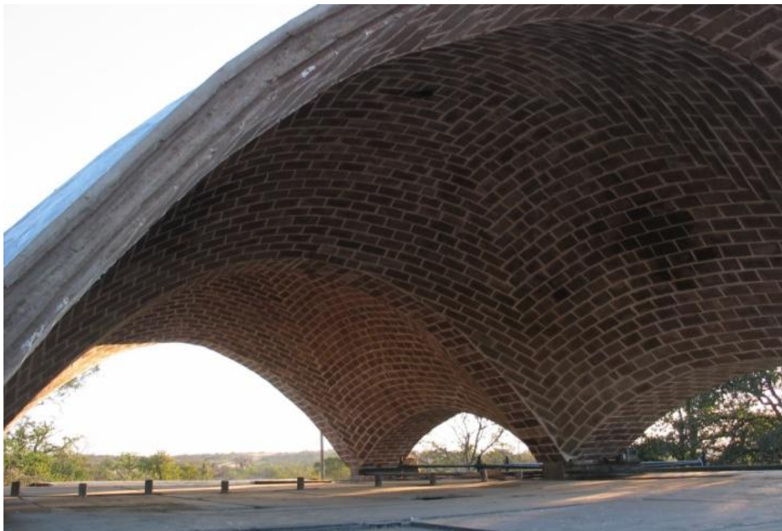
Figure 3 Showing part of the completed Mapungubwe Interpretation Centre
